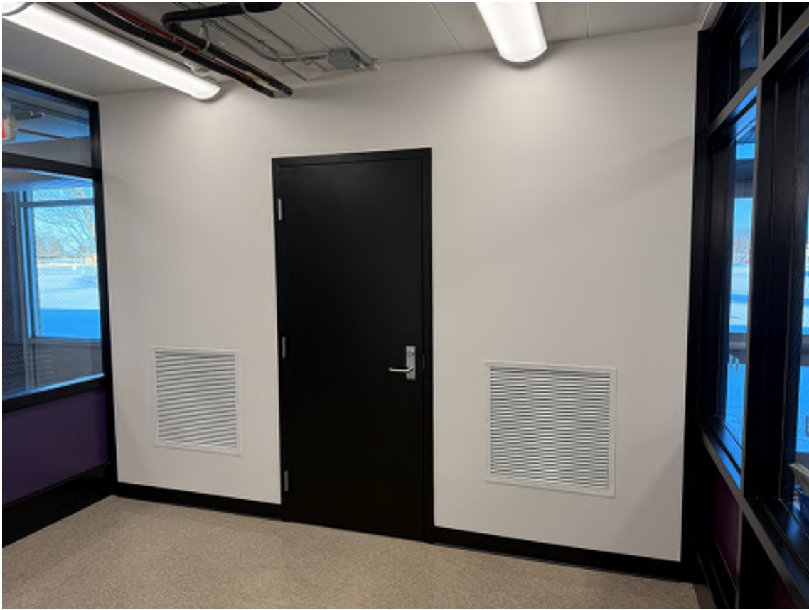
Double VUV enclosure between classrooms after completion.
