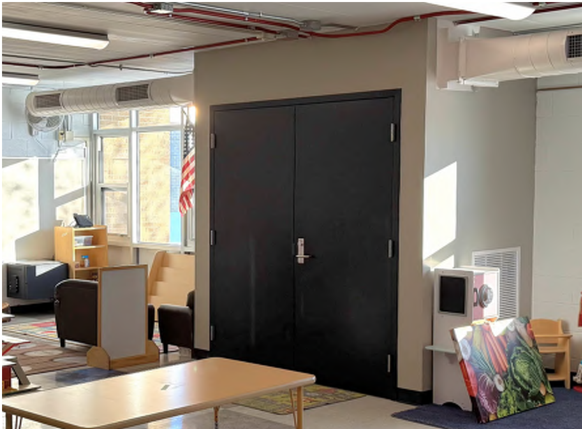
Single VUV enclosure in classroom after completion.
