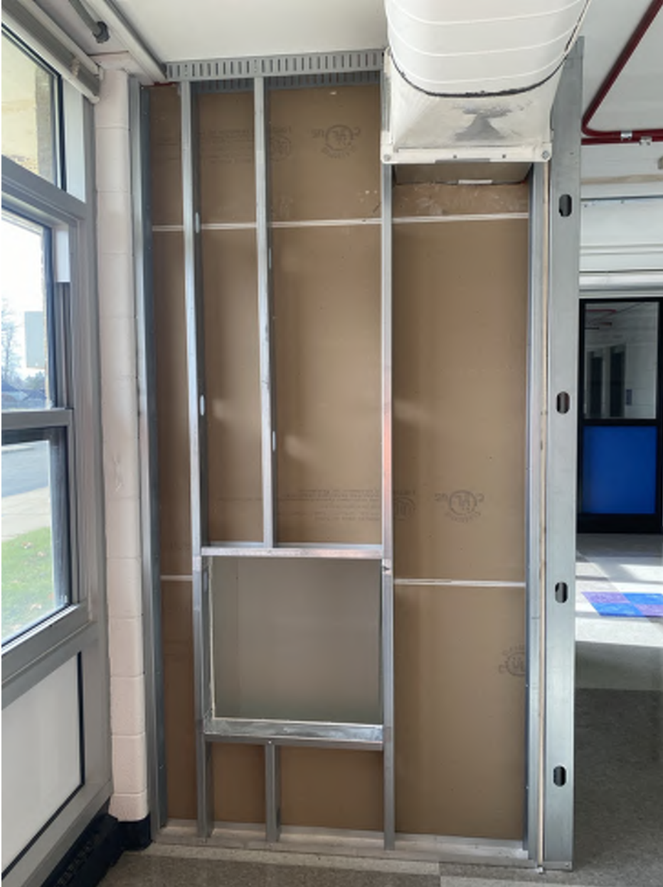
Wall framing prior to boarding the other side at a single VUV enclosure.
