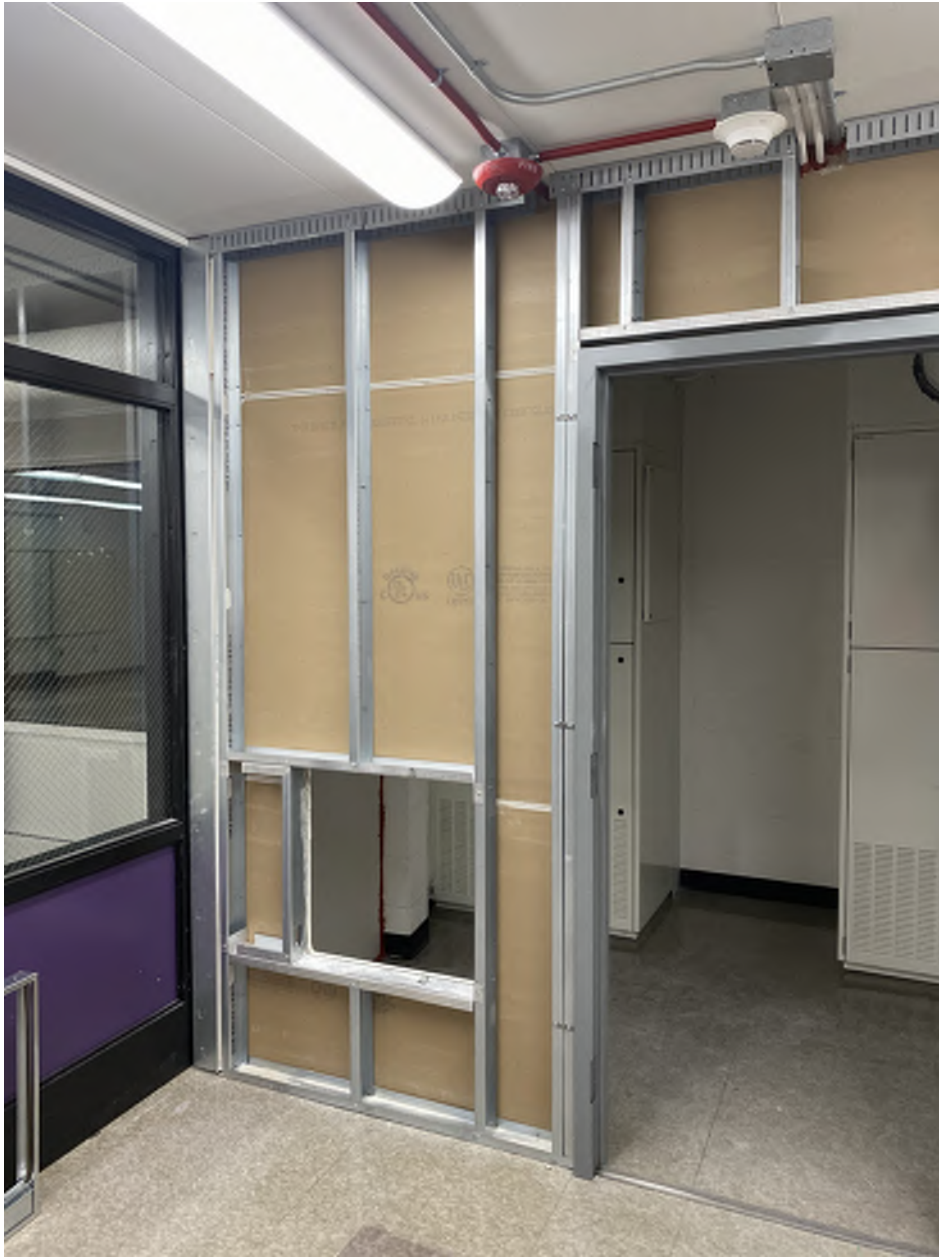
Left and right sides of the wall framing at a double VUV enclosure. Double VUV enclosures are located in the work rooms between classrooms.
