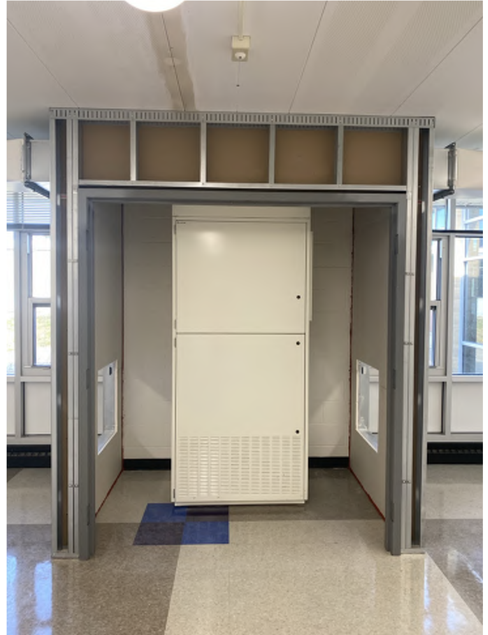
Wall framing in progress at a single VUV enclosure located in a classroom.
