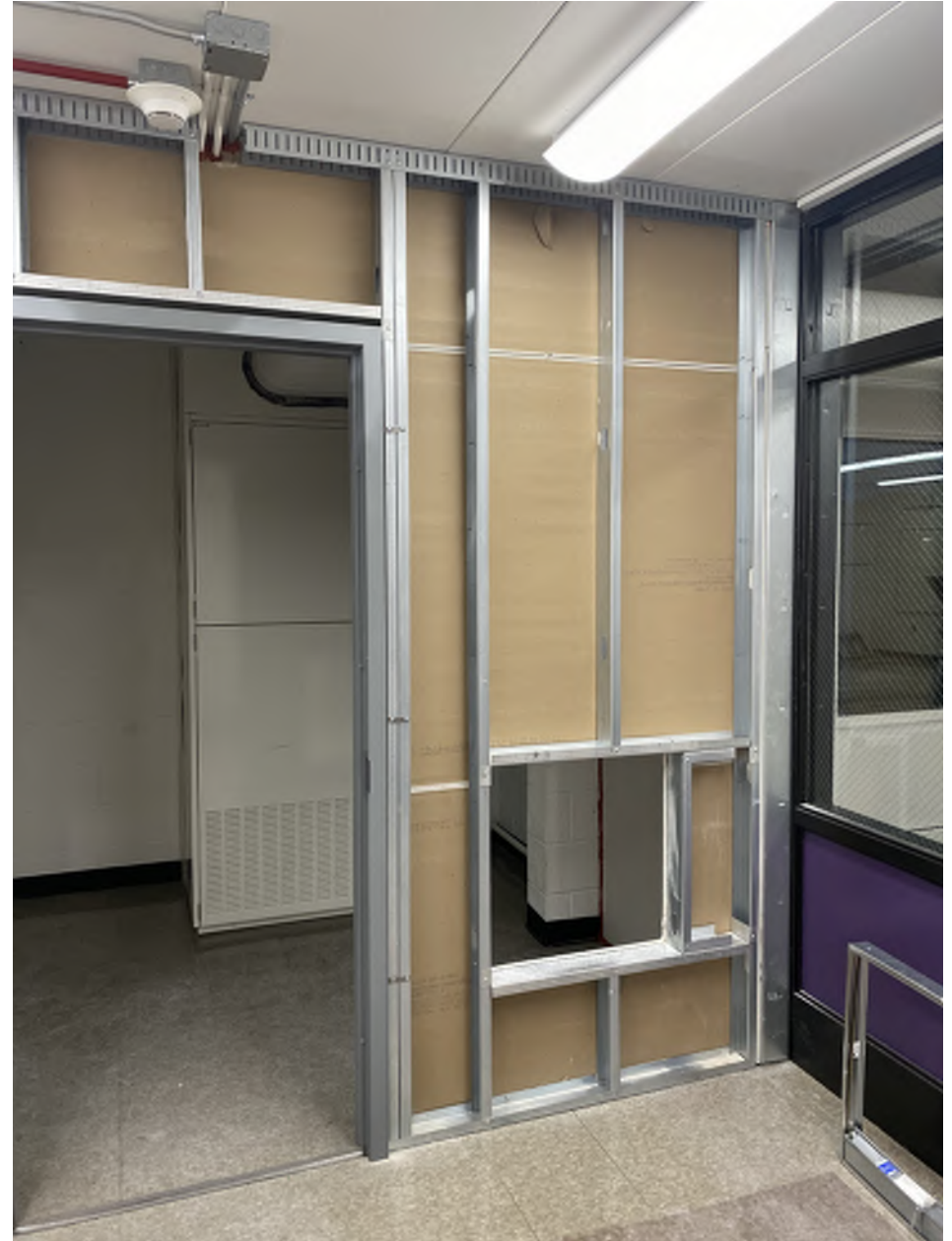
Left and right sides of the wall framing at a double VUV enclosure. Double VUV enclosures are located in the work rooms between classrooms.
