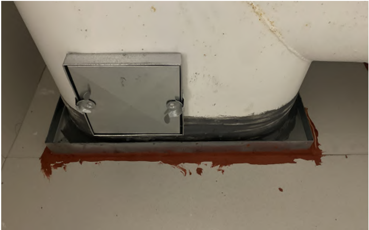
Access door installed in VUV enclosure duct.
