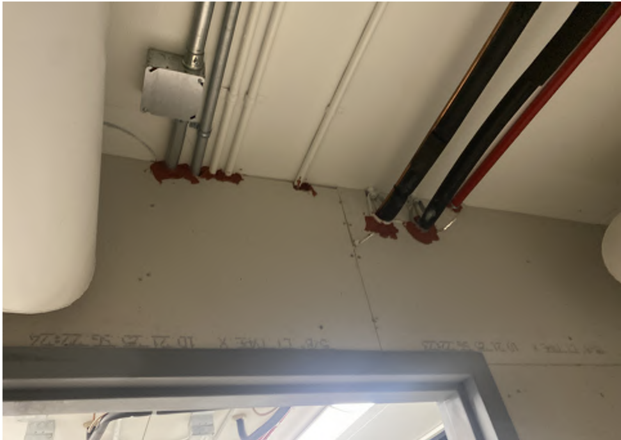
Fire caulking around raceways going through VUV enclosure wall.
