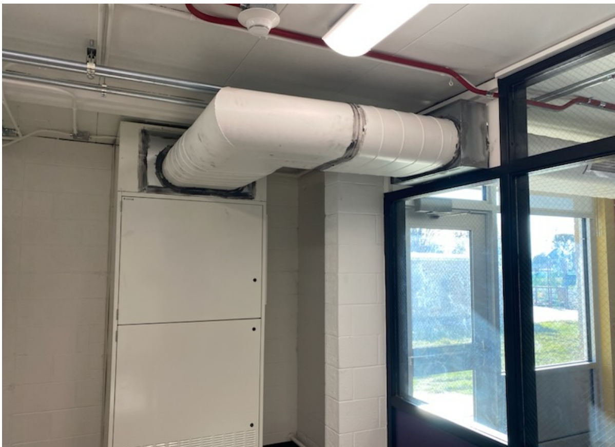
Supply duct damper installed in a workroom for the VUV enclosures.
