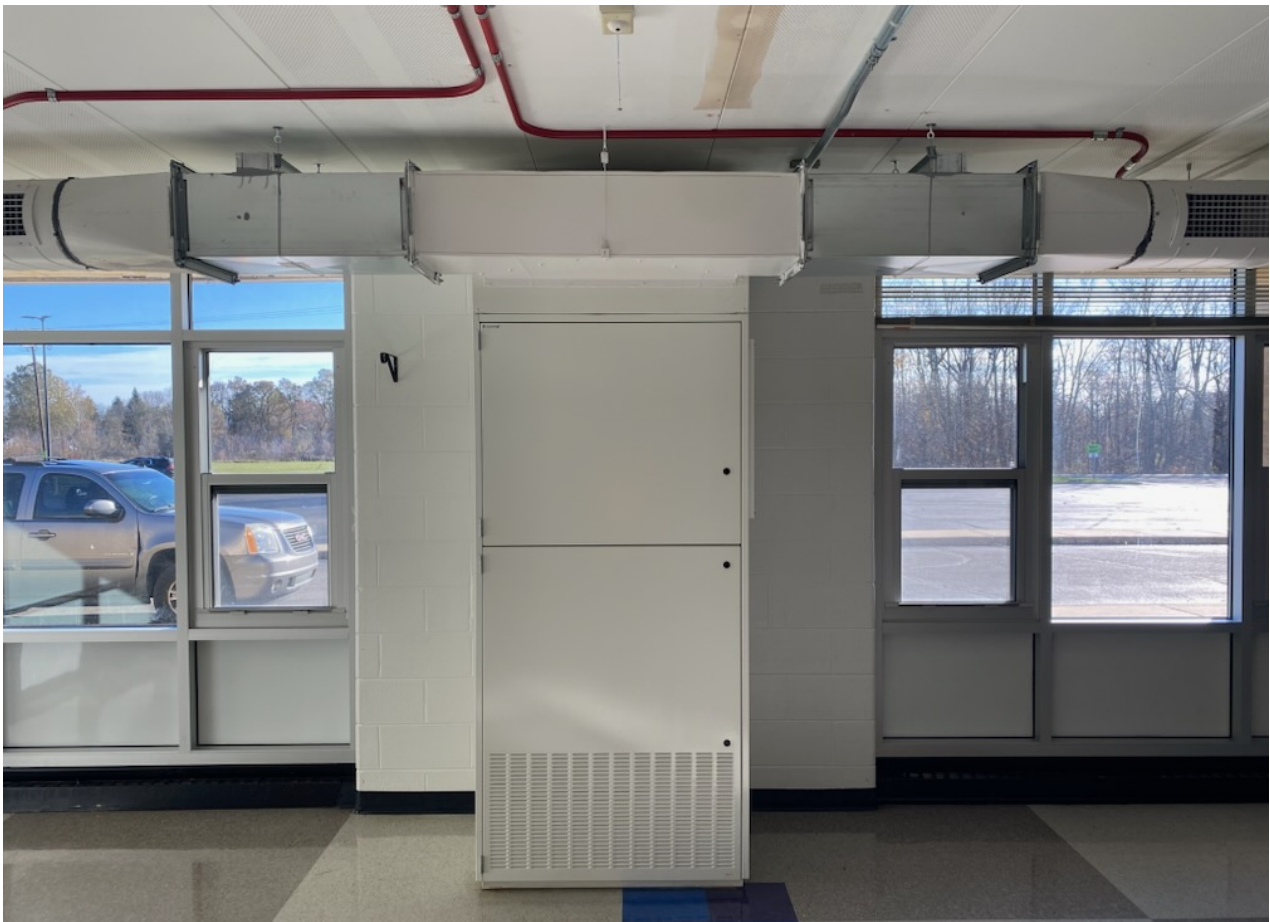
Rectangular supply duct extended to prepare for VUV enclosure construction in a classroom.
